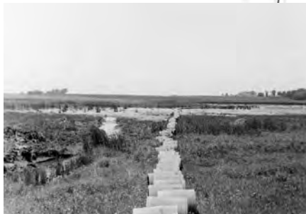
Installation of subsurface tile for wetland drainage in Iowa, circa 1950. Photo courtesy of USFWS.
