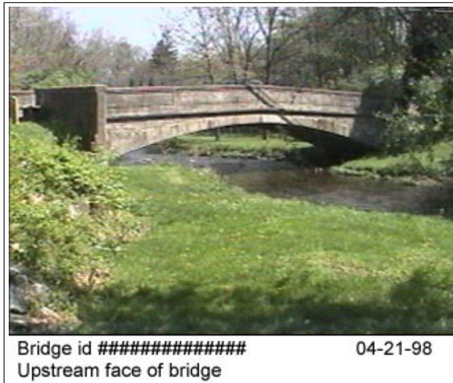
Figure 7. Video image of upstream face of field-viewed bridge.
