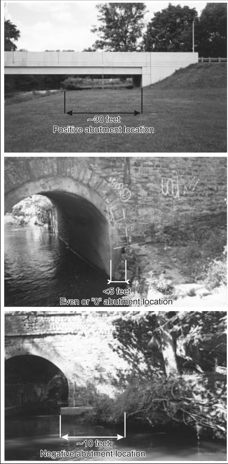
Figure 21. Abutment location.
