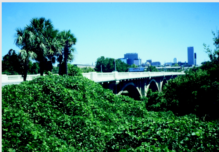
Shallow ground water in the Columbia, S.C., metropolitan area contains a variety of volatile organic compounds, but mostly at low concentrations.
