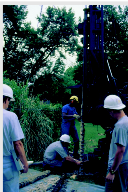
Shallow wells for the urban ground-water study were installed by the U.S. Geological Survey with assistance from the South Carolina Geological Survey.
