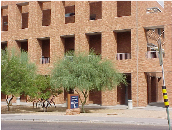
USGS building on the University of Arizona campus, home of Arizona USGS state office, shared with other agencies.
