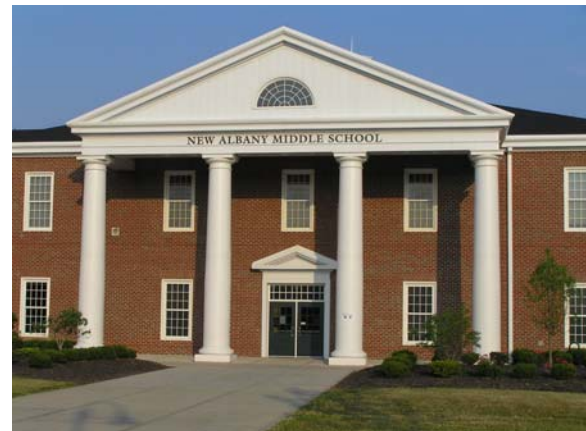
GeoTech Ohio, held at New Albany Middle School, provided not only an excellent building facility for such an event, but also a 120-acre campus, including protected woodland, wetland, prairie, and lake for conducting field research. It was one of the best places that I have ever taught.
