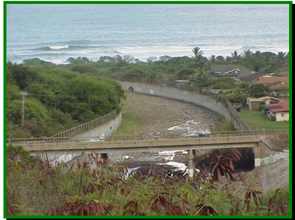
The mouth of Iao Stream as it flows into the Pacific Ocean on the north side of Wailuku. The stream's channelization affects water quality, runoff, and ocean marine life. The width of the channel gives some indication of the tremendous volume that this and other streams experience during significant precipitation events.
