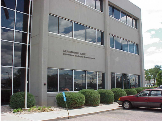
The USGS MESC building in Fort Collins.
