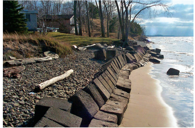
Figure 15. Armored shoreline on Lake Ontario that disrupts natural coastal processes and generally results in accelerated erosion.
