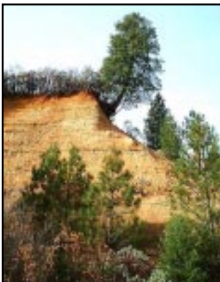
Physical hazards at hydraulic mine sites include highwalls (left photo) and open shafts (right photo). Highwalls are steep unstable slopes subject to sudden collapse. Shafts vary from tens to hundreds of feet in depth and connect with horizontal mine workings including drift mines and drainage tunnels.
