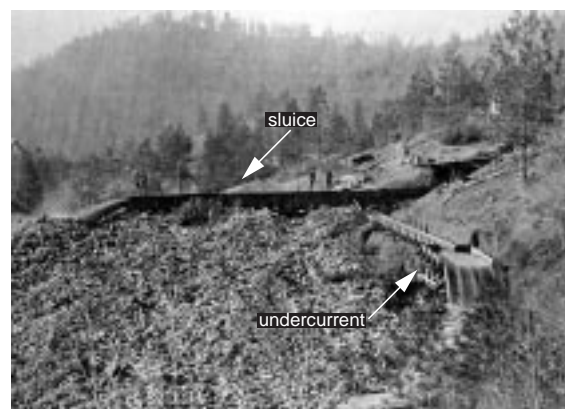
Figure 6. Undercurrent in use, circa 1860, Siskiyou County, California.
