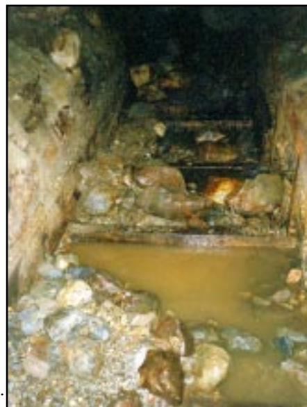
Tunnel sluice with mercury-contaminated sediments.
