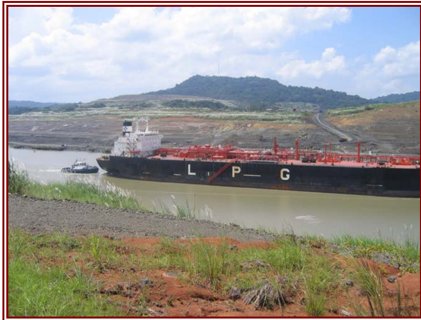
FIGURE 4-9: TUGBOAT ACCOMPANIES TRANSIT TANKER AT CULEBRA CUT NEAR LA PITA SUR MODERNIZATION CONSTRUCTION SITE
