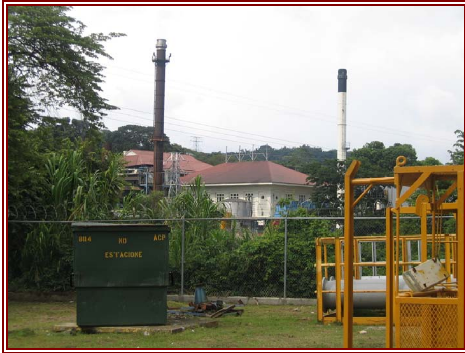
FIGURE 4-8: THERMO-ELECTRICAL POWER PLANT AT MIRAFLORES
