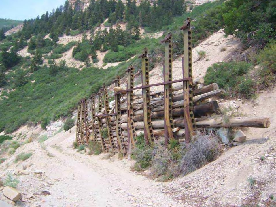
In two different areas, steel cribbing has been installed to stabilize the talus slopes. Some of the steel crib beams are strongly bent, indicating downslope movement of loose talus behind the cribs. If the cribbing should fail, the mine road could be blocked and substantial repair could be required to reopen the road.
