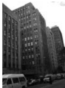
Figure 5.31. New York Presbyterian Hospital.
