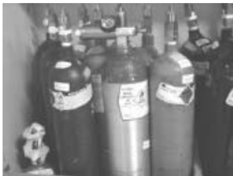
Figure 5.8. Color-coding and pin-indexed connectors for medical gas tanks.
