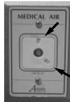
Figure 3.4. A typical pin-indexed medical air outlet. The pins on the regulator fit into the holes at 12 and 5 o'clock. Each gas regulator has a 12 o'clock pin and one other pin.
