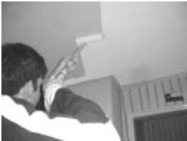
Figure 6.46. This paint is pink when applied, but will be white when it dries.
