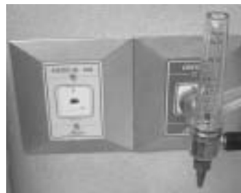
Figure 5.10. The holes for the pins are located at 12 o'clock and 5 o'clock. Also, the oxygen outlet is green, and the medical air outlet is yellow.
