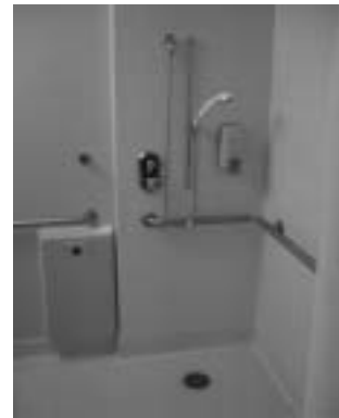
Figure 5.45. A shower with handrails.
