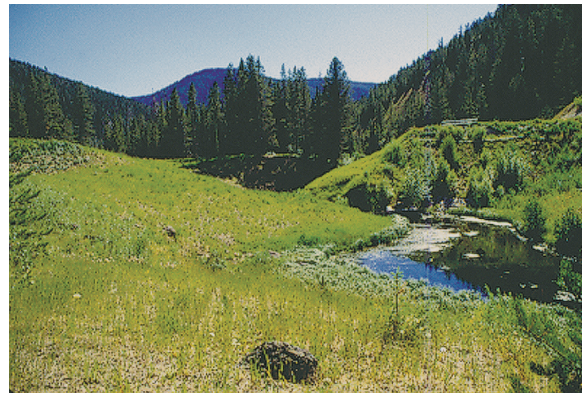
Figure 41. The remains of Mystic Lake Dam, a small water-supply dam in southwestern Montana, United States, which was constructed in 1903–04 on the site of a landslide dam. The earthfill dam was purposely breached in 1984 because of the hazard it posed to the downstream city of Bozeman. Photograph taken in 1997.
