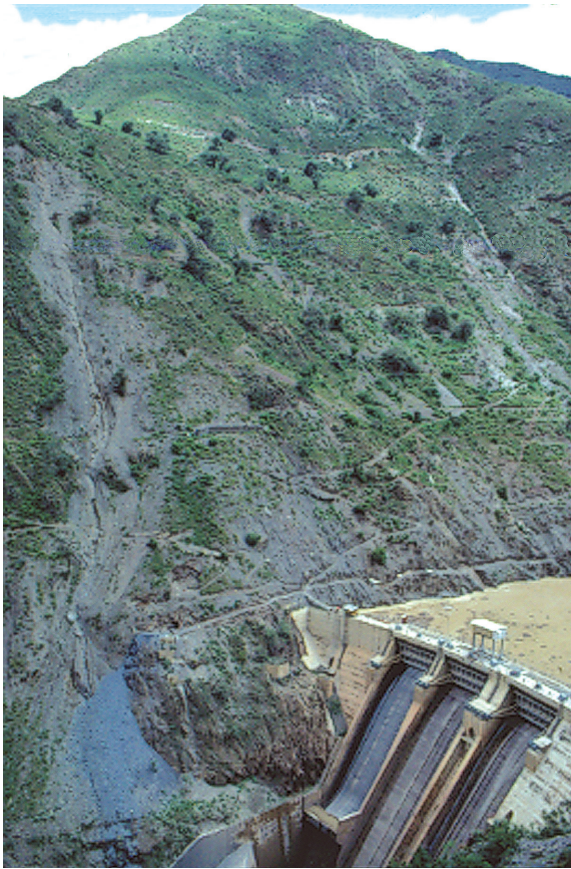
Figure 12. Looking upstream at the right-abutment landslide at Tablachaca Dam, Peru. Photograph taken in 1982.
