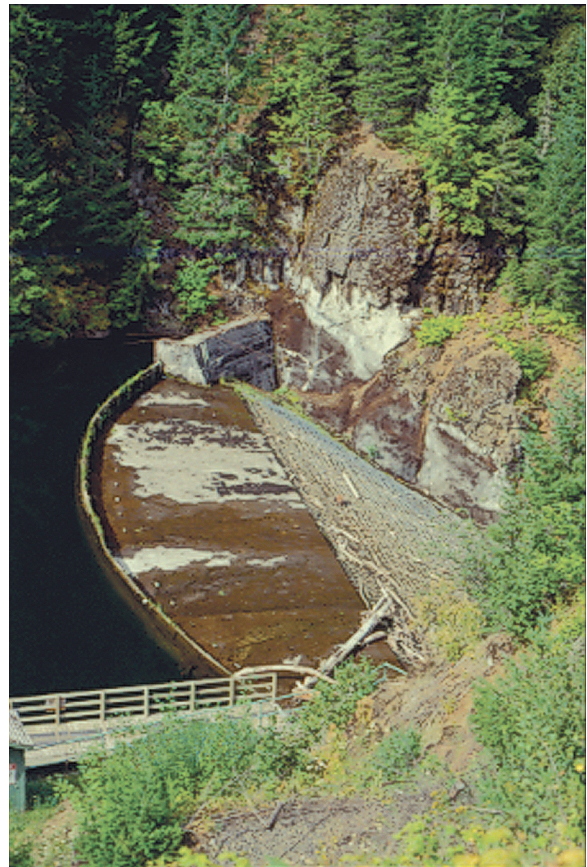
Figure 14. Lake Harriet Dam, Cascade Range, Oregon, United States. The basalt that forms the left abutment of this dam is part of the reactivated toe of a 50-km 2 landslide mass. Photograph taken in 1999.
