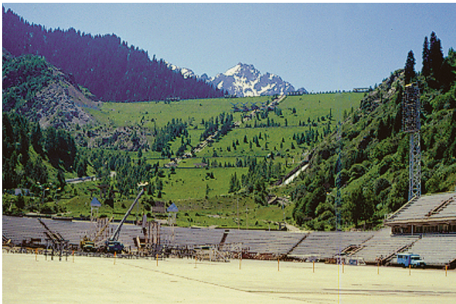
Figure 31. Medeo Dam, a debris-flow retention structure on the Malaya Alma-Atinka River in Kazakhstan, which is founded on debris-flow deposits. Photograph taken in 2001.
