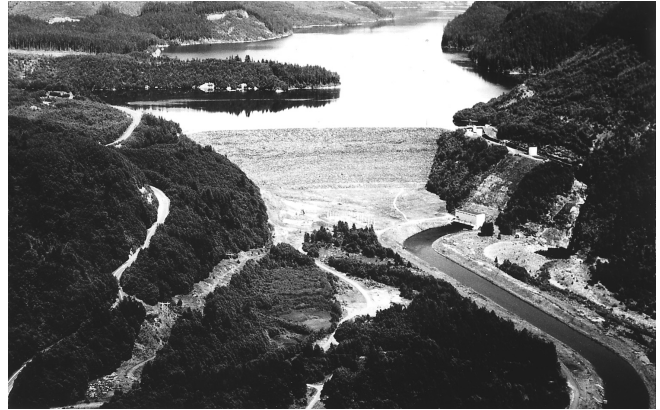
Figure 27. Aerial view of Swift Dam, Lewis River, western Washington State, United States, showing forested debris-flow deposits that form the right abutment of the dam (see fig. 28). Photograph by Lynn Topinka, U.S. Geological Survey.
