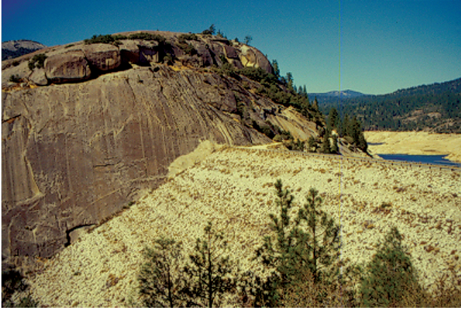
Figure 2. Mammoth Pool Dam, San Joaquin River, California, United States. Note the exfoliation sheets and blocks in the granodiorite that forms the right abutment. Photograph taken in 1998.
