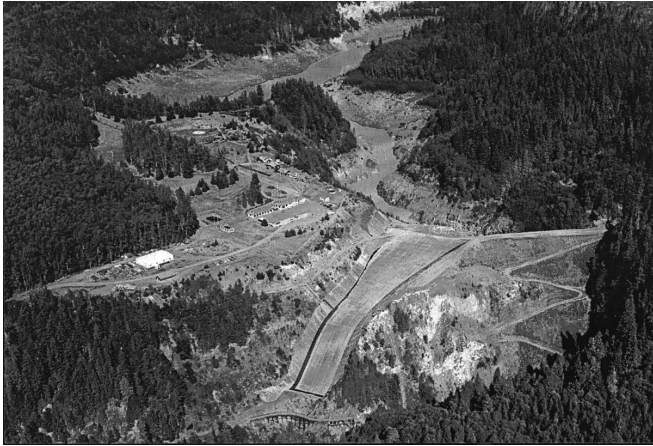
Figure 25. Aerial-oblique view of Mud Mountain Dam, western Washington State, United States. At both banks of the White River, the dam abuts into a Pleistocene mud-flow (lahar) deposit from Mount Rainier volcano. Photograph taken in 1979 by U.S. Army Corps of Engineers.
