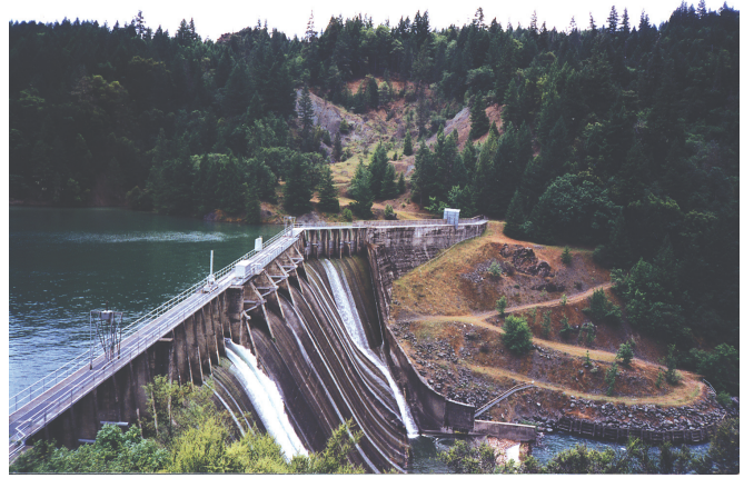
Figure 38. Scott Dam on the Eel River, northern California, United States. During construction in 1921, the left end of this dam was diverted downstream to miss the landslide on the left bank of the river, resulting in a “dogleg” in the dam. Photograph taken in 1997 by J.C. Gamble, Pacific Gas and Electric Company, San Francisco.
