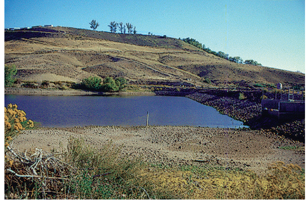
Figure 19. Fruitgrowers Dam, an irrigation dam in western Colorado, United States, showing apparent landslide topography in shale of the left abutment. Photograph taken in 1999.
