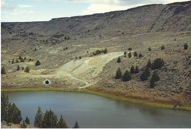
Figure 35. Star Mountain Dam, a 21-m-high irrigation dam in southeast Oregon, United States. The right abutment of this dam is the toe of a large landslide. After the dam failed in 1983 due to flood erosion of the unlined spillway at the landslide right abutment, a circular concrete-lined spillway was installed within the embankment. Photograph taken in 1998.
