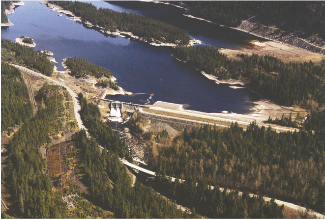
Figure 23. Oblique aerial view of Cheakamus Dam, British Columbia, southwestern Canada. The foundation of the dam is mainly Rubble Creek Wash, a debris avalanche–debris flow deposit (see fig. 24). Photograph taken in 1999 by BC Hydro, Burnaby, British Columbia.
