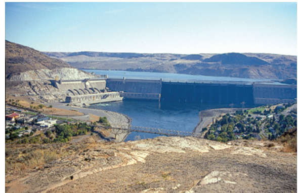
Figure 21. Grand Coulee Dam, eastern Washington State, United States. In 1969, the original landslide-prone glacial-soil right abutment was removed to make room for the second powerplant at the right end of the dam (left edge of photo). Photograph taken in 1999.
