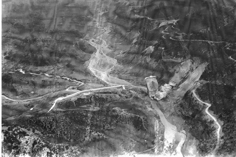
Figure 7. Looking upstream at the remains (center of photograph) of St. Francis Dam, southern California, United States, soon after its 1928 failure, which resulted in a catastrophic flood that killed about 450 people. The failure began in the toe of a large prehistoric landslide that formed the left abutment (right side of photograph); note fresh landslide scarps. Photograph taken in 1928, courtesy of Department of Geography, University of California at Los Angeles.
