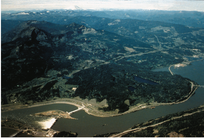
Figure 16. Oblique aerial view of Bonneville Dam in the Columbia River Gorge, Washington and Oregon, United States. The right (Washington) abutment is the toe of the huge Bonneville landslide, which is the most recently active part of the Cascades landslide complex. Photograph by Derek Cornforth, Landslide Technology, Portland, Oregon.
