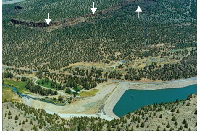
Figure 36. Oblique-aerial view of Ochocho Dam, central Oregon, United States, and the huge rock slide–lateral spread that serves as its right abutment. Note the long head scarp (marked by arrows) of the slide along the upper part of the ridge. Photograph taken in 1999 by U.S. Bureau of Reclamation.
