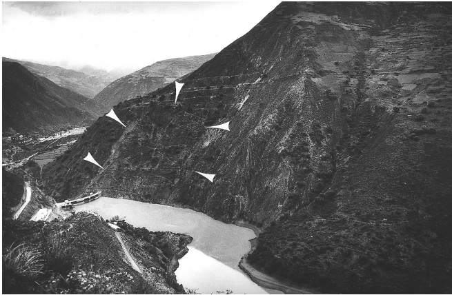
Figure 11. Oblique view of Tablachaca Dam, Peru. The pre-existing rock slide in the right abutment is outlined by arrows. This slide was reactivated in the 1970s, probably because of infiltration from the reservoir. Photograph taken in 1982.
