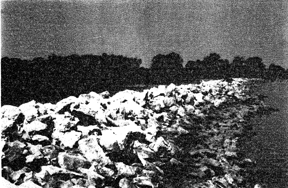
Figure 9. Rip-rap dike separating Lake Erie (right) from Darby Marsh (left); this wetland is part of the Ottawa National Wildlife Refuge (August 1982).
