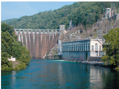
Tapoco Project, Cheoah Dam
