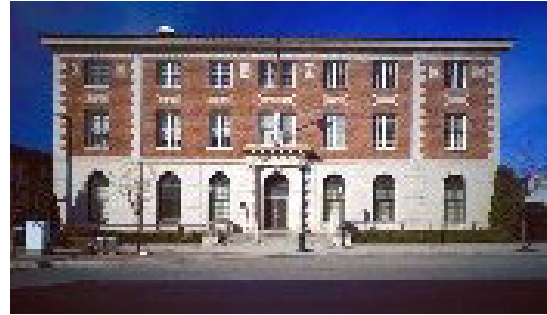
The Federal Building in Coeur d'Alene, Idaho is one of many with ENERGY STAR labels
