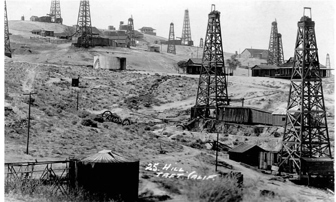
Figure 3.52. Drilling and production activity at Twenty-five Hill near Taft, California. Note the dense well spacing. Photograph courtesy of Don Arnot, West Kern Oil Museum.
