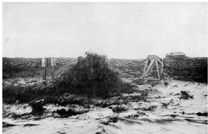
Figure 3.34. A dam of sandbags was built around the Lakeview 1 well. This photograph was taken on October 2, 1910. Photograph by W.C. Mendenhall in Pack (1920).
