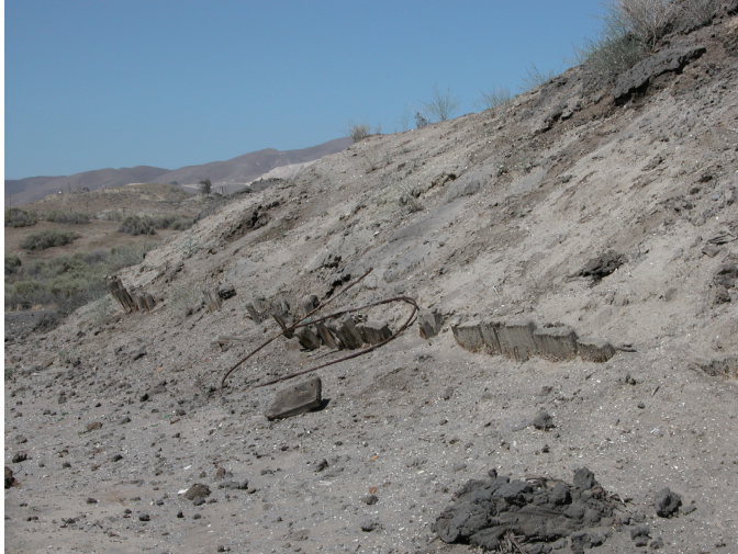
Figure 3.37. Remnants of the embankment built to contain the Lakeview gusher. Note the pieces of sandbags in the lower right.
