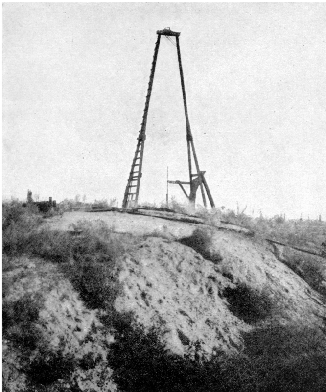
Figure 3.12. Very early derrick used to drill shallow wells that supplied the Jewett and Blodgett asphalt refinery in the 1890s. See also figure 3.11. Photograph from Pack (1920).
