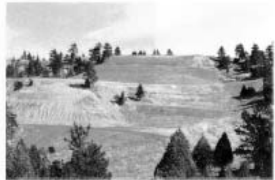
C. Slope reduction and installation of waterbreaks completed
