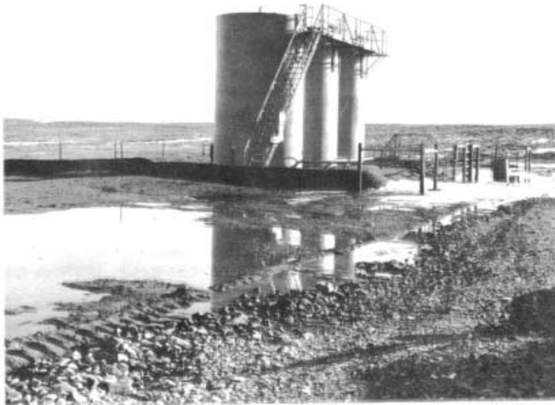
PHOTOGRAPH 5. TYPICAL PRODUCTION FACILITY FIREWALL
