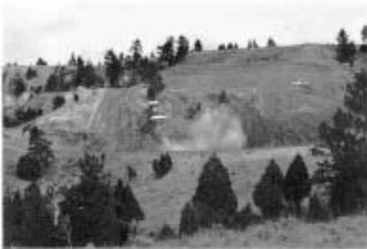
B. Slope reduction on the well site.
