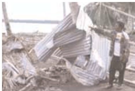
Figure 22. Damage caused by the tsunamis that hit Papua New Guinea on July 17, 1998. Photograph by Guy Gelfenbaum, USGS.
