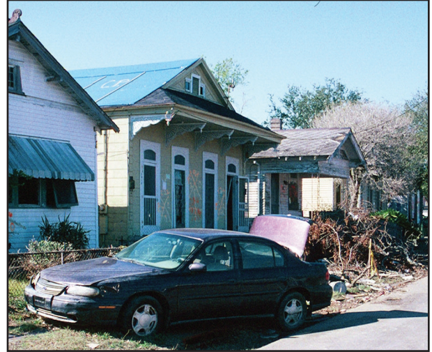
Flood-damaged houses, New Orleans
