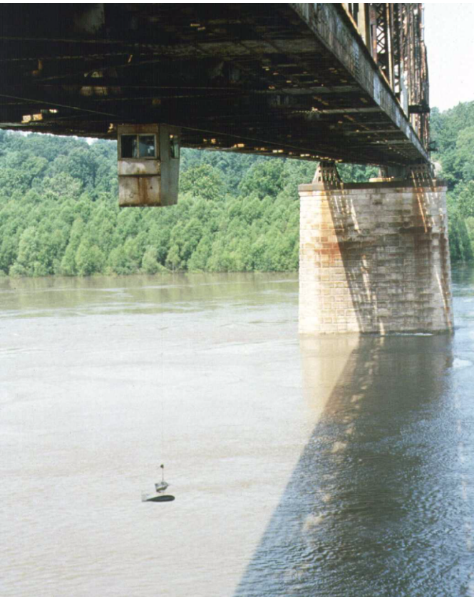
Figure 1. U.S. Geological Survey (USGS) personnel measuring flow at the Mississippi River at Thebes during the 1993 flood (USGS personnel are in the monorail system, located below the bridge deck, lowering the flow meter and 300-pound weight by cable to the river.)
