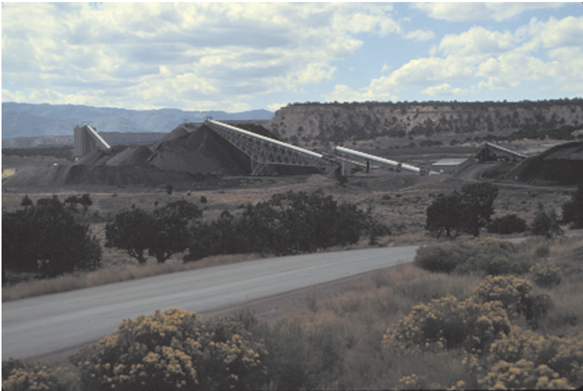
Photograph. Darrah Siding loadout in the northern part of the Wasatch Plateau.
