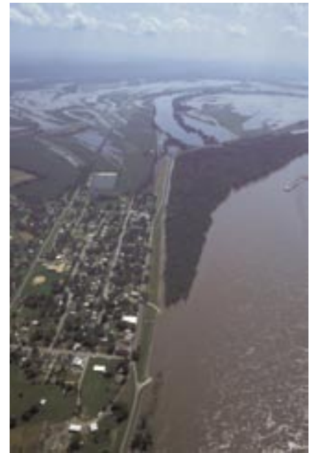
Grand Tower, Illinois, during the height of the flooding along the Mississippi River. Photo by Kevin Oberg, USGS.
