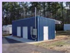
A building was constructed on-site at EPA Athens and outfitted with instruments to measure moisture content and soil gas pressure at several depths beneath and outside the footprint of the structure.
