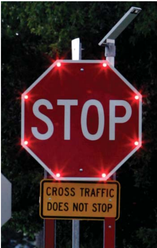
A red light flashes on each corner of this stop sign at the intersections of Ohio 49 and Ohio 707 in rural Mercer County, Ohio, on Sept. 26, 2006. The flashing lights on the stop sign allow it to be seen from greater distances, even in daylight. The intersection had been the scene of numerous accidents. To improve traffic safety without busting their budgets, states are installing the cable barriers, painting distance dots on roads to discourage tailgating and placing stop signs that light up like Christmas trees at dangerous intersections. (AP Photo/Al Behrman)
