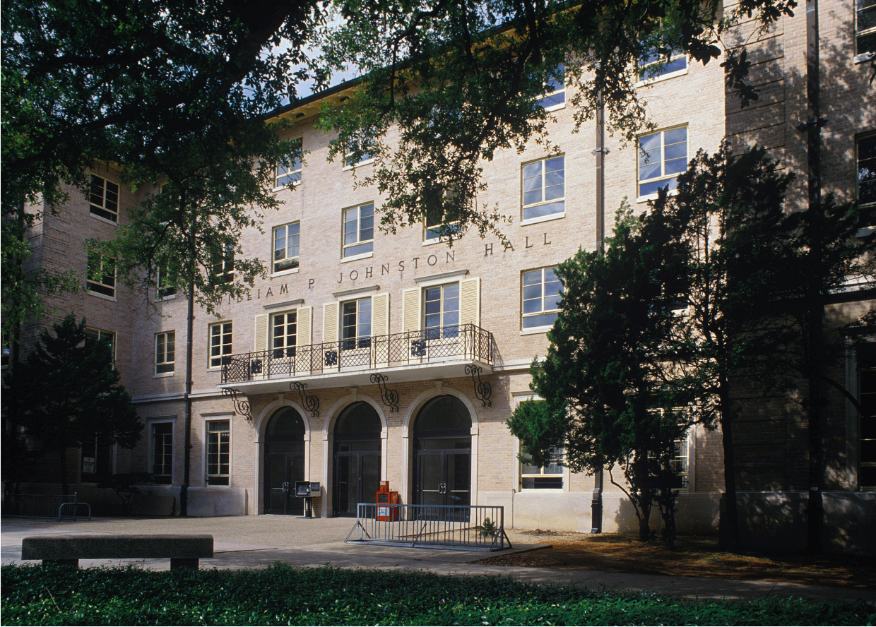
Figure 4 - Johnston Hall, Site of Hurricane Katrina Fraud Task Force Command Center
