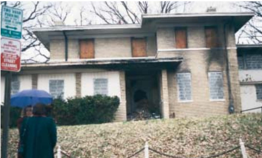
The chancery of Liberia before restoration.
