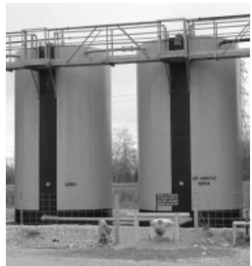
Figure 11. Unlabeled flammable condensate storage tanks, CJ Waller lease.
