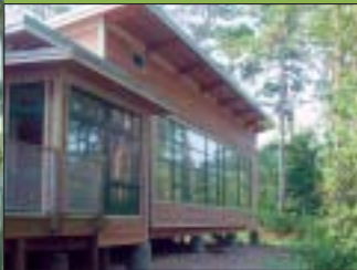
The indoor environment is enhanced further through abundant daylight and fresh air ventilation.
