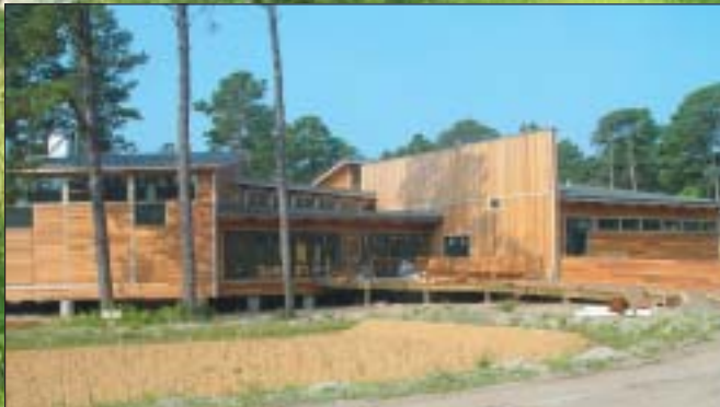
The Center uses an innovative constructed wetlands wastewater treatment system. The system includes a primary clarifier, a subsurface-flow-constructed-wetland with recycle, and a re-circulating sand filter. The effluent is used to flush toilets.
