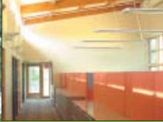
Recycled, renewable, and non-toxic building materials such as bamboo floors, cedar walls, and recycled carpet provide good indoor air quality.
