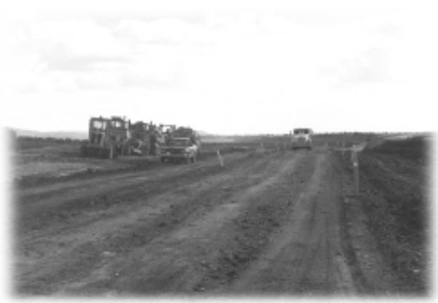
Road construction on Northern Cheyenne Reservation (photo by Teri Peterson).
