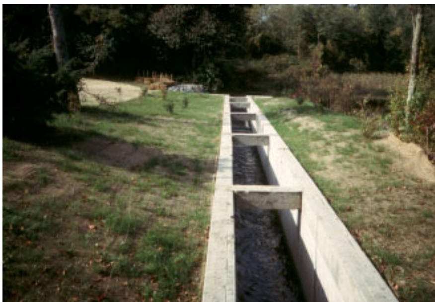
This fishway on the Mashpee River restored alewife and blue-backed herring access to spawning sites in Mashpee Pond, upstream of a barrier dam. USFWS photo.
