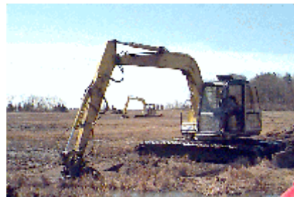
Excavators working at the East River saltmarsh restoration site.
