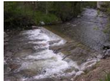
In-stream concrete barrier
