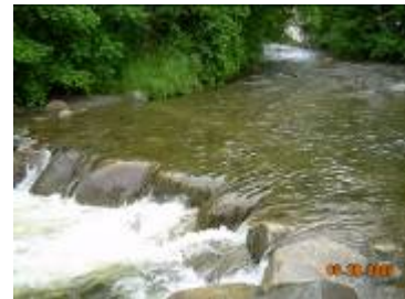
Barrier after weir construction
