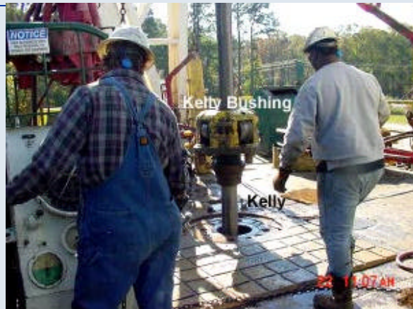
Fig. 15. Lowering kelly bushing
