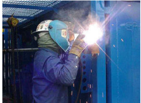
Fig. 1. Welding with fire control
