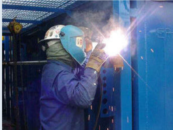
Fig. 3. Welding - hot work
