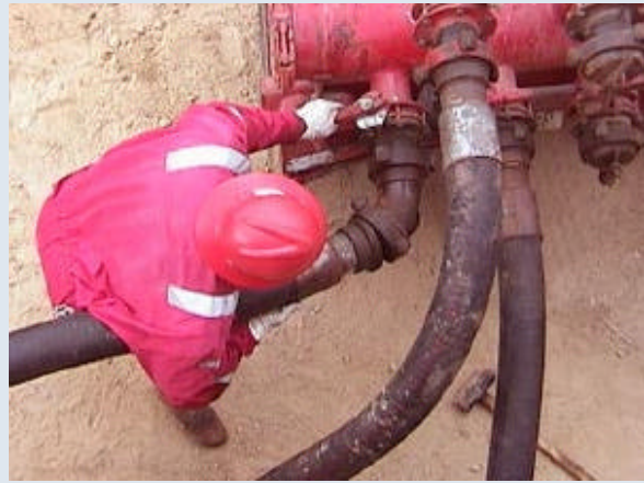
Fig. 13. Connecting blender up to manifold
