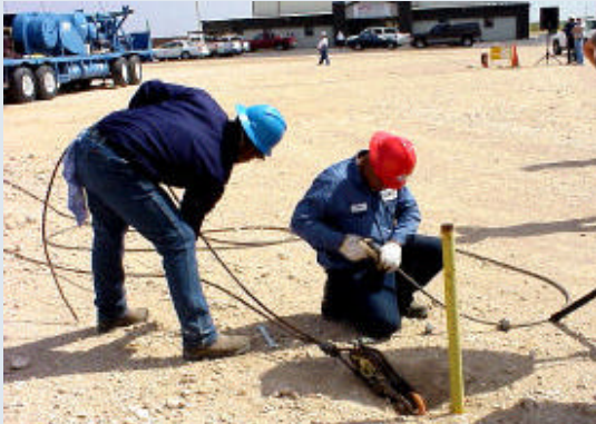
Fig. 6. Installing guy line anchor
