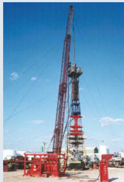
Fig. 21. Snubbing rig with blow out preventer (BOP)
