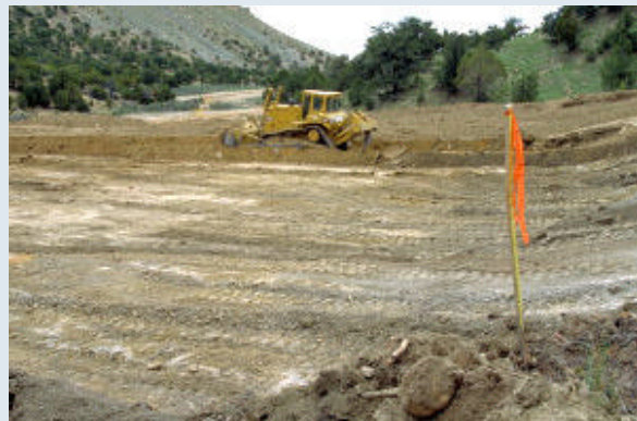
Fig. 4. Excavating at a drill site
