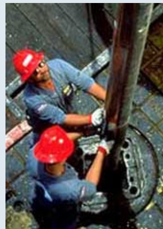
Fig. 4. Installing production casing
