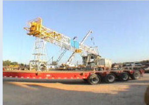
Fig. 6. Rigging up the mast
