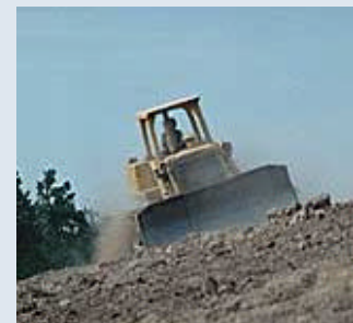
Fig. 2. Leveling uneven ground
