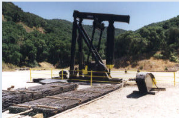
Fig. 10. Assembling beam pumping unit
