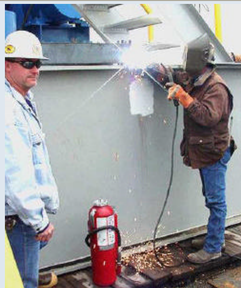
Fig. 2. Welding with fire control
