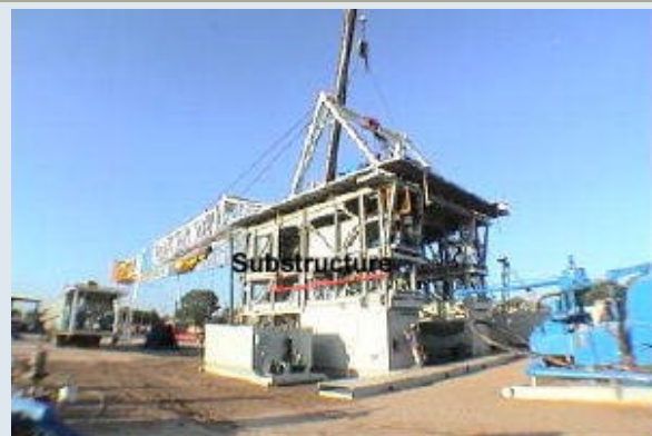
Fig. 2. Setting up the substructure
