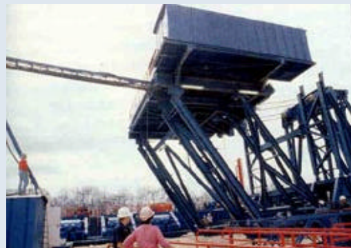
Fig. 3. Raising the doghouse and rig floor
