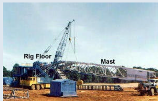
Fig. 4. Setting mast on rig floor
