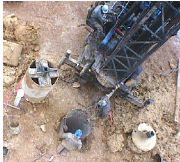
Fig. 1. Conductor hole
