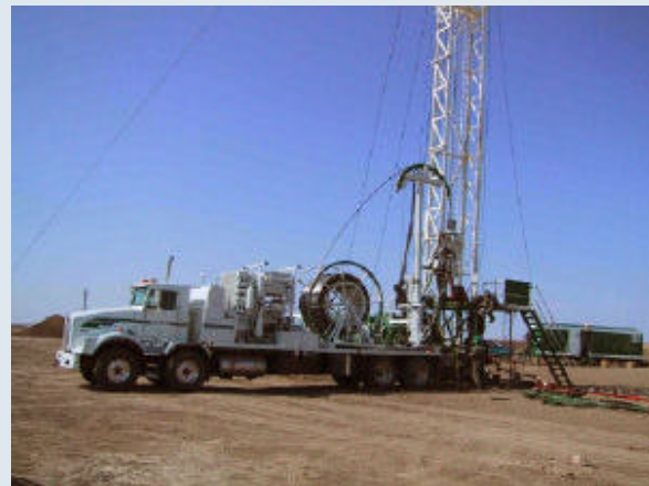
Fig. 7. Installing coil tubing
