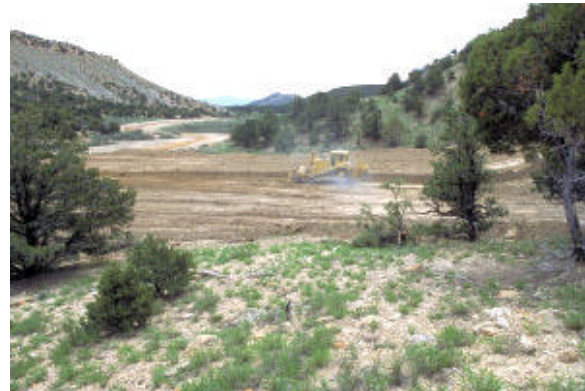
Fig. 1. Clearing the drilling site
