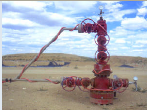
Fig. 3. Wellhead on flowing well
