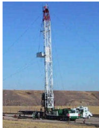
Fig 2. Well completion service rig
