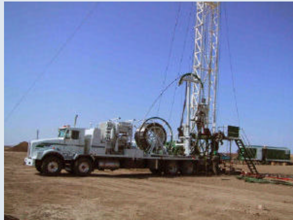
Fig. 22. Installing coil tubing
