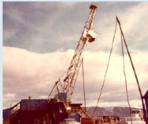
Fig. 7. Raising the mast
