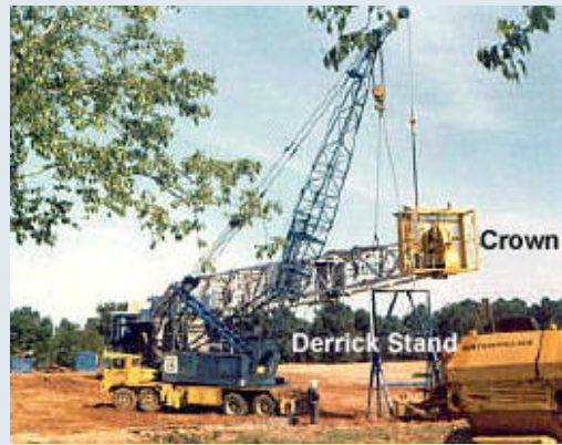
Fig. 5. Setting crown on derrick stand
