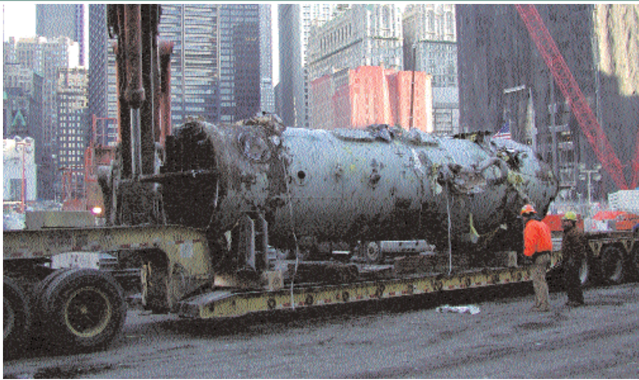
Freon tank being removed from the site.
