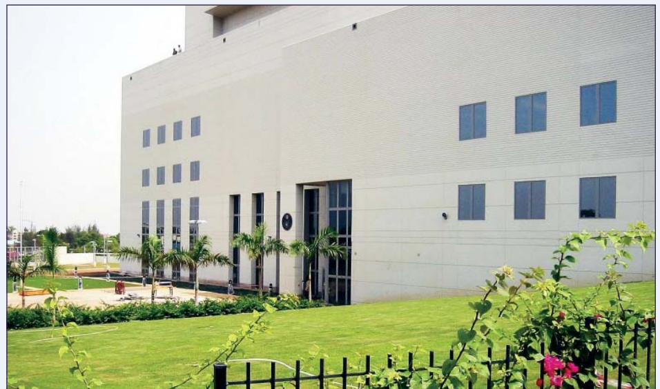
The new U.S. Embassy Compound, Abuja, Nigeria State Department Photo
