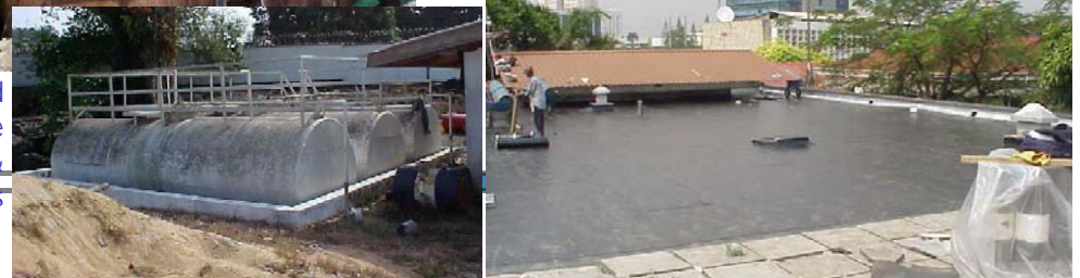
Underground Fuel Storage Tank Upgrades & Replacements
