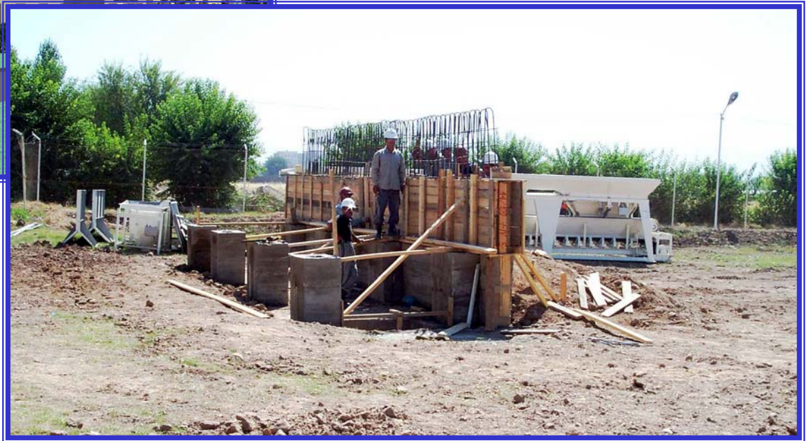
Construction photo of Dushanbe, Tajikistan NEC
