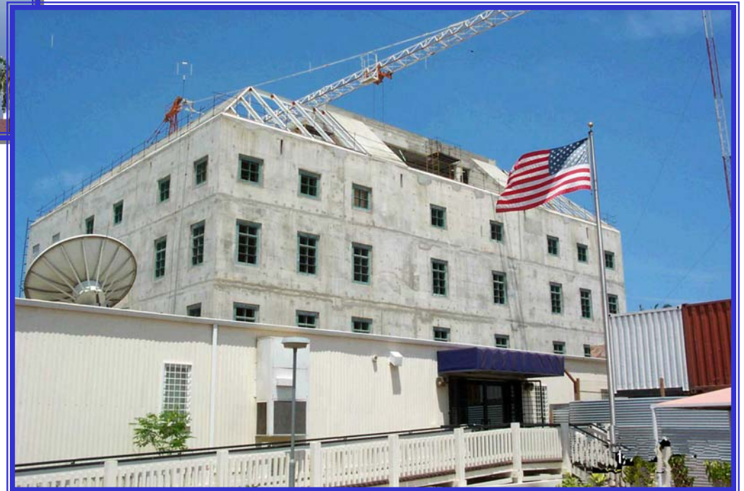
Construction photo of Luanda, Angola NEC
