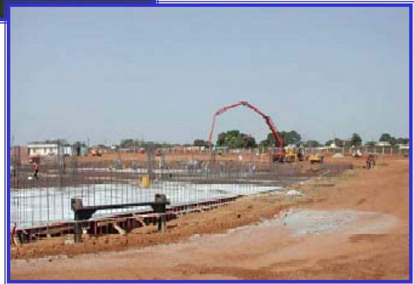
Construction photo of Conakry, Guinea NEC
