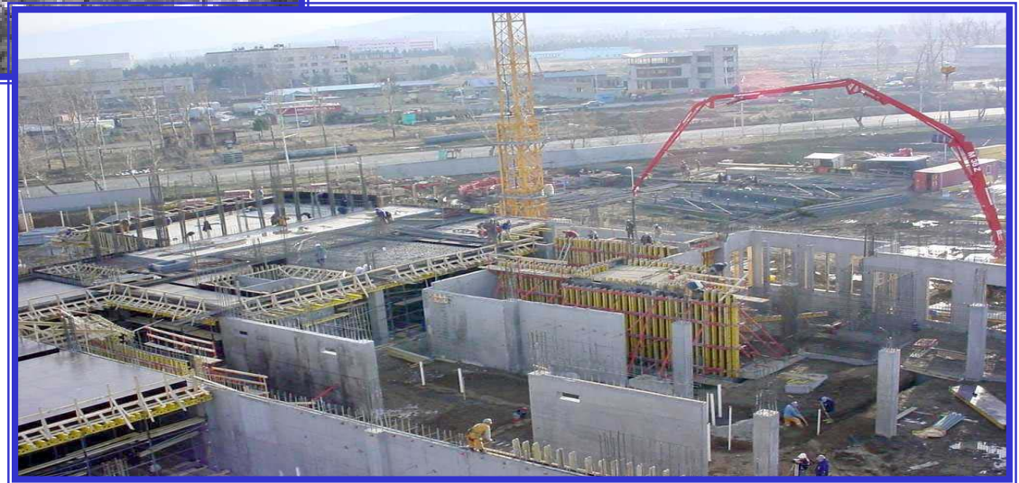
Construction photo of Tbilisi, Georgia
