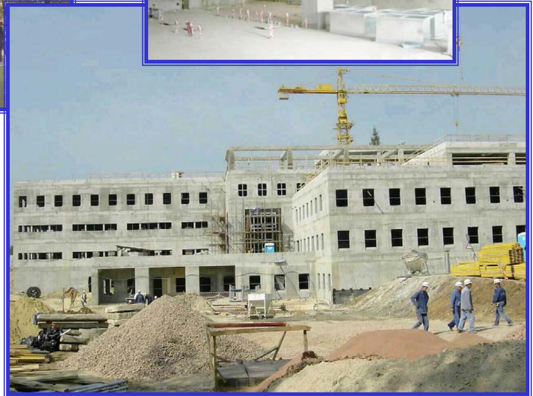
Construction photos of Sofia, Bulgaria NEC
