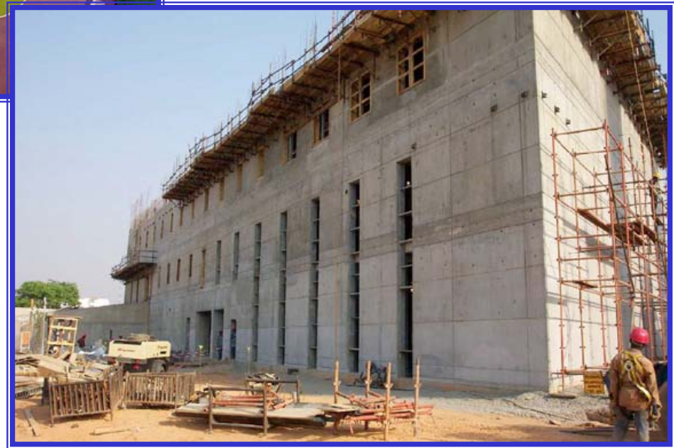
Construction photo of Abuja, Nigeria NEC
