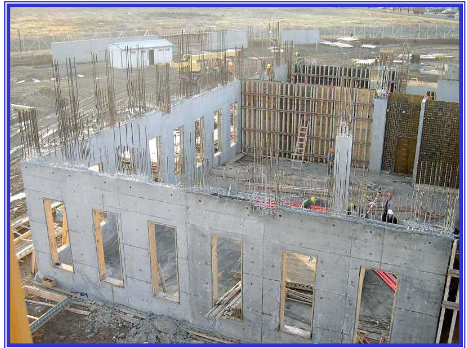
Construction photo of Tashkent, Uzbekistan NEC
