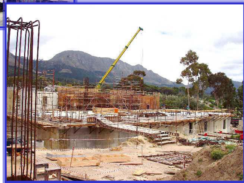
Construction photo of Cape Town, South Africa NEC
