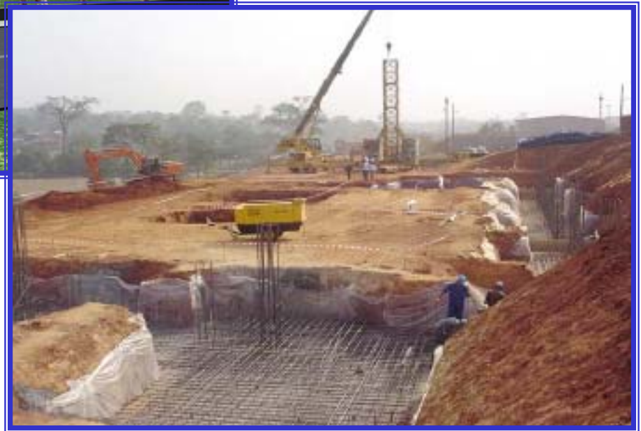
Construction photo of Yaounde, Cameroon NEC
