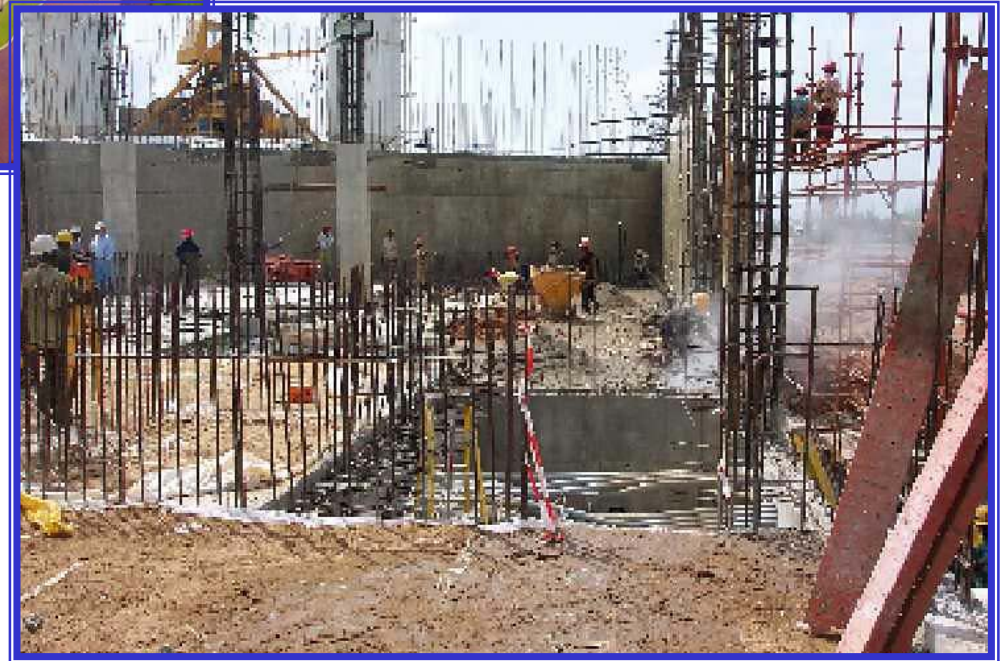
Construction photo of Abuja, Nigeria NEC 36% Complete
