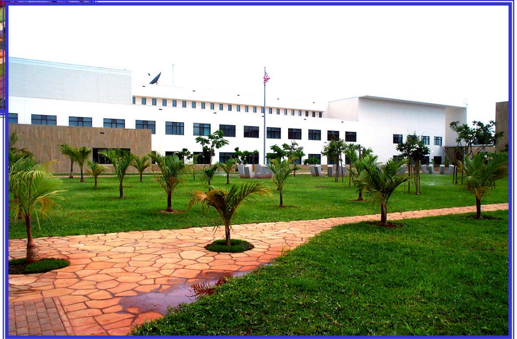
Photograph of Dar es Salaam, Tanzania NEC 100% Complete
