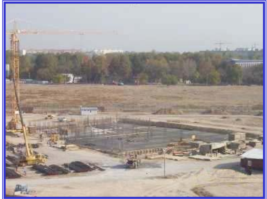
Construction photo of Tashkent, Uzbekistan NEC 19% Complete
