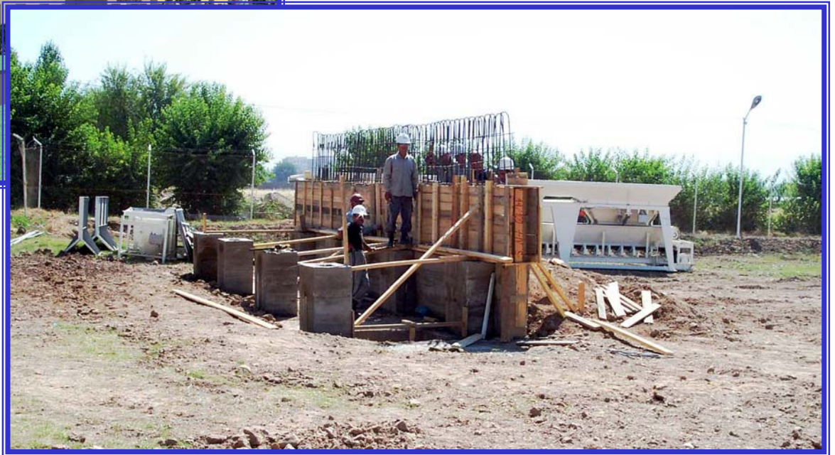
Construction photograph of Dushanbe, Tajikistan NEC 25% Complete
