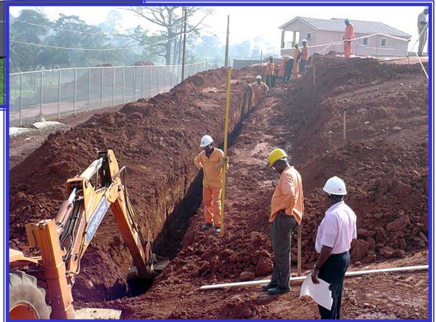
Construction photo of Yaounde, Cameroon NEC 19% Complete
