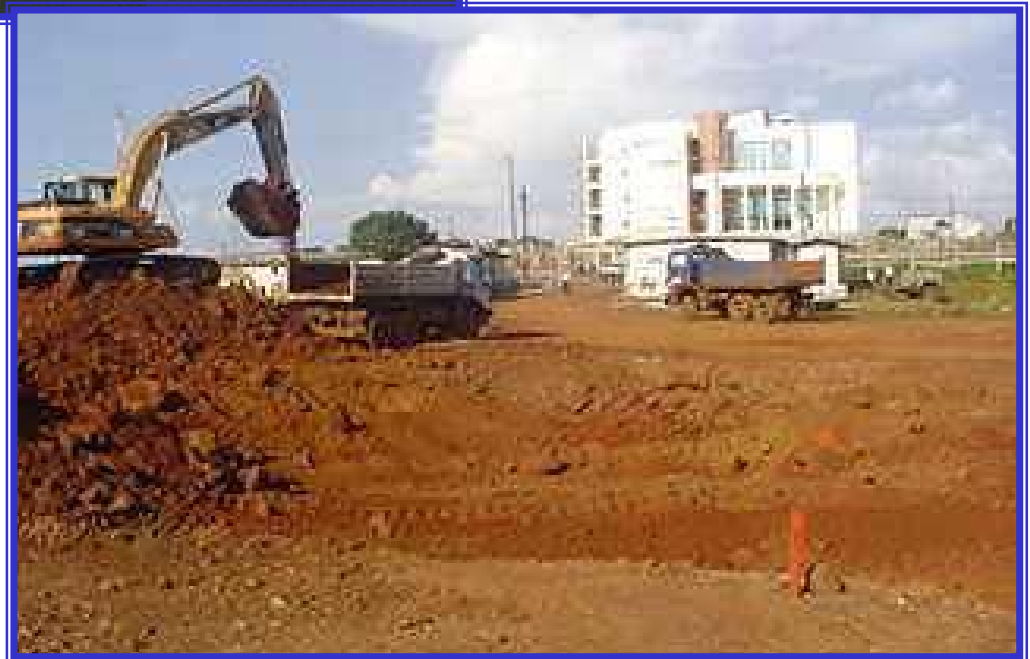
Construction photo of Conakry, New Guinea NEC 16% Complete
