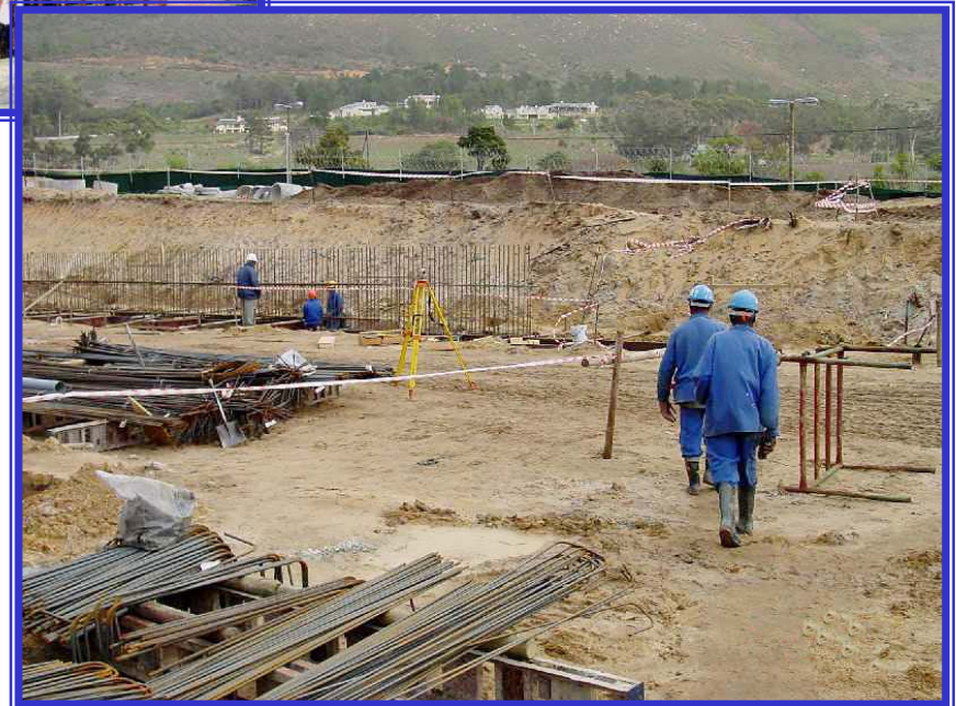
Construction photo of Cape Town, South Africa NEC 20% Complete
