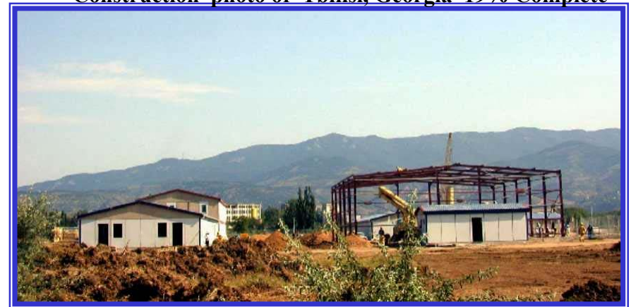
Construction photo of Tbilisi, Georgia 19% Complete
