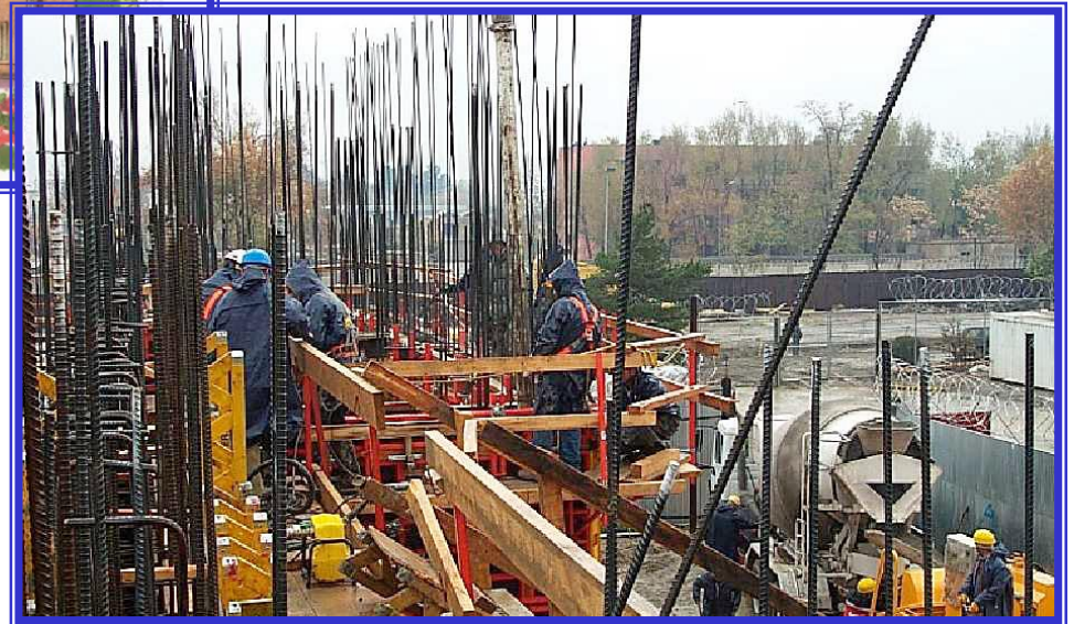
Construction photo of Kabul, Afghanistan NEC (Phase 2) 33% Complete
