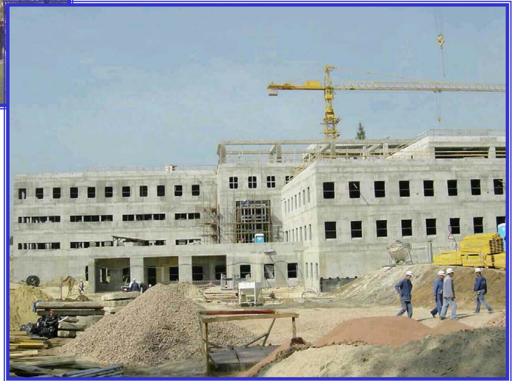
Construction photo of Sofia, Bulgaria NEC 39% Complete
