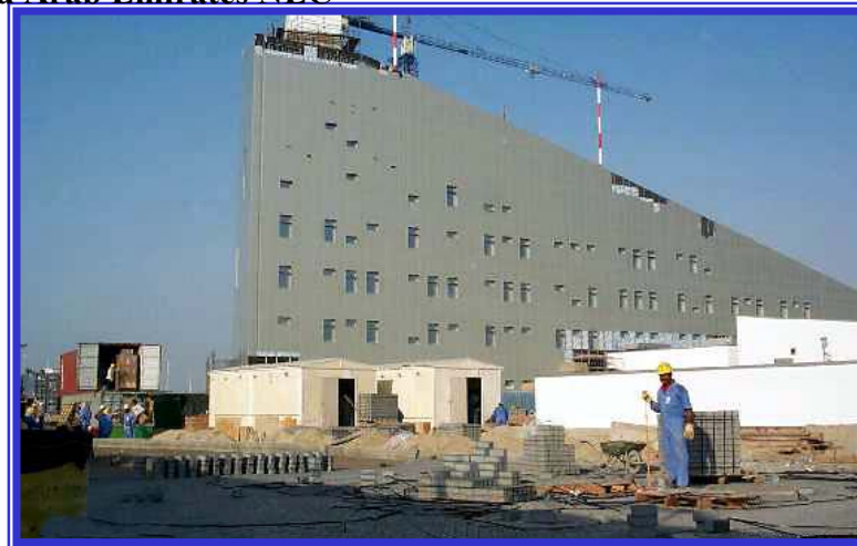
Construction photo of Abu Dhabi, United Arab Emirates NEC 90% Complete
