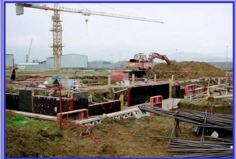
Construction photo of Tbilisi, Georgia 19% Complete
