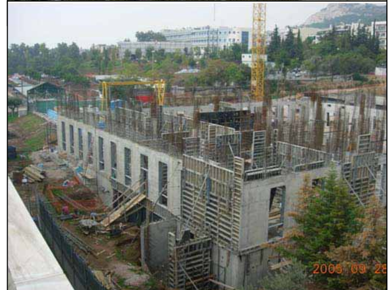
28,000sf Extensive Green Roof Athens, Greece
