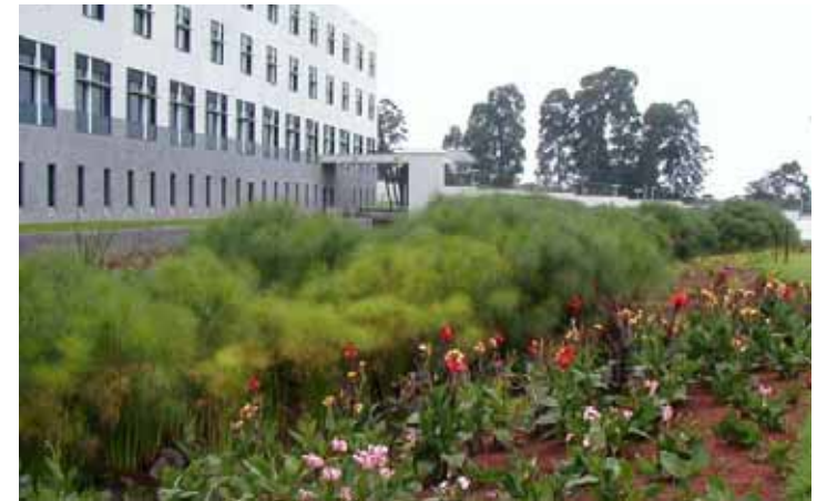
Constructed Wetland Nairobi, Kenya
