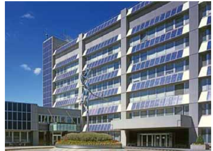
OBO's Photovoltaic Installation Geneva, Switzerland
