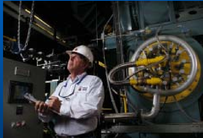
Above: Operations Engineer in JFRC Boiler Room
