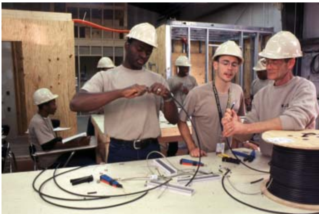
A Job Corps electrical systems technical instructor trains students on proper methods and tools for preparing coaxial cable for installation.
