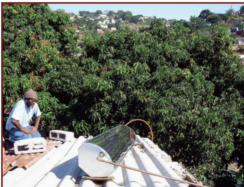
A local official in the Durban area of South Africa found low-cost solar water heating simple enough that he installed it on his own.
