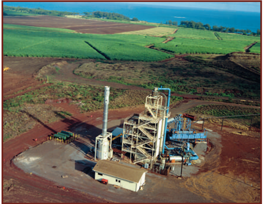
The Pacific International Center for High Technology Research operates this biomass gasification demonstration project located in Hawaii. This gasification plant will initially process bagasse from the neighboring sugarcane refineries, but is designed to receive a wide variety of biomass.
