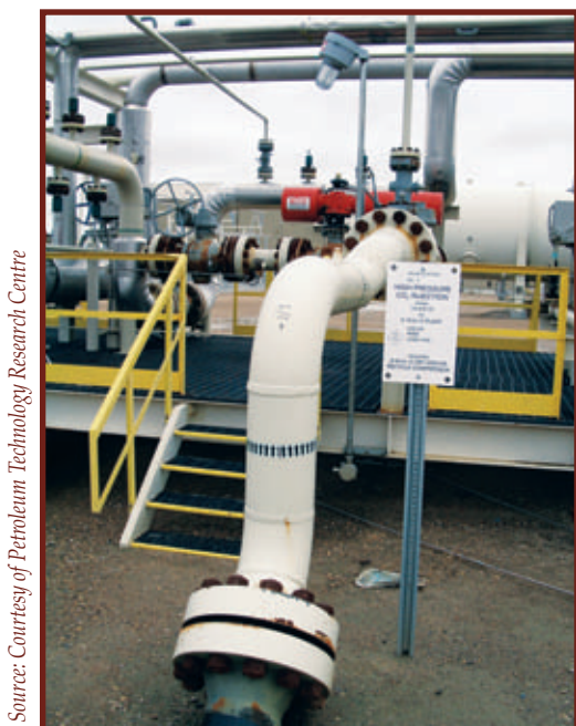
Carbon dioxide enters the Weyburn field from the Great Plains Synfuels Plant near Beulah, North Dakota. The gas travels 205 miles through a carbon steel pipeline and will be sequestered in an underground storage facility. Projects like this will comprise the Carbon Sequestration Leadership Forum.
