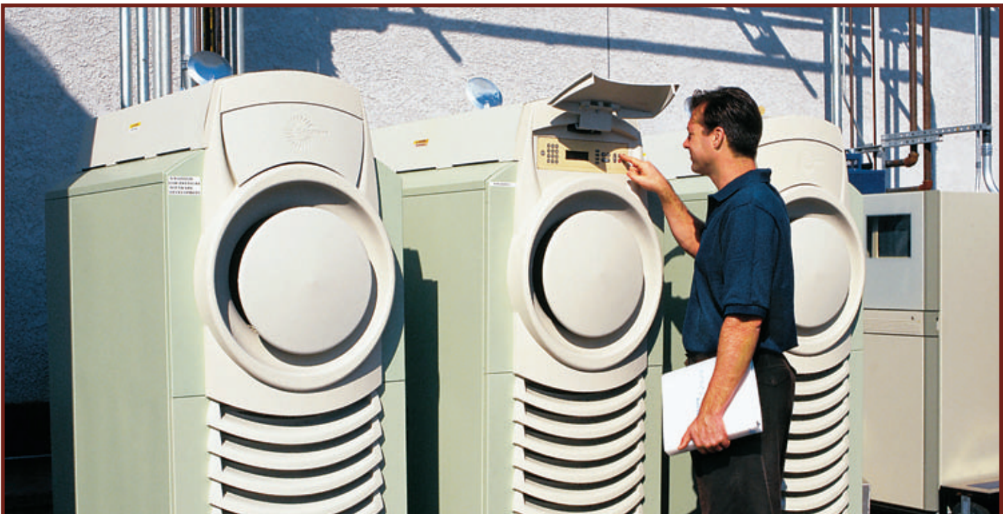
The EPA implements voluntary programs that promote profitable opportunities for reducing emissions of methane, while creating profitable activities for the coal, oil and natural gas, landfill, and agricultural industries. Pictured above are three microturbines powered by landfill methane.
