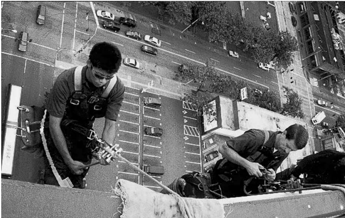
Washington DOSH Window washers using rope descent system and boatswain.
