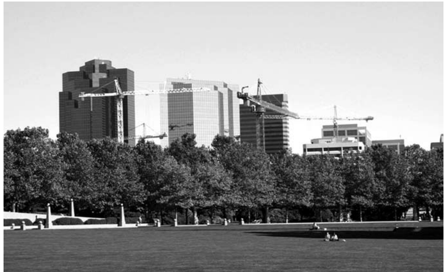
Washington DOSH Construction is booming in downtown Bellevue.
