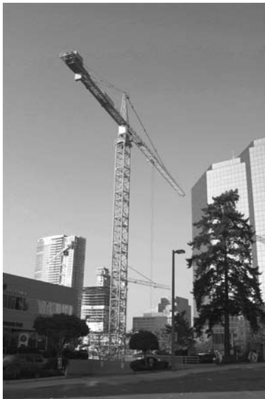
Washington DOSH Tower crane at work in downtown Bellevue.
