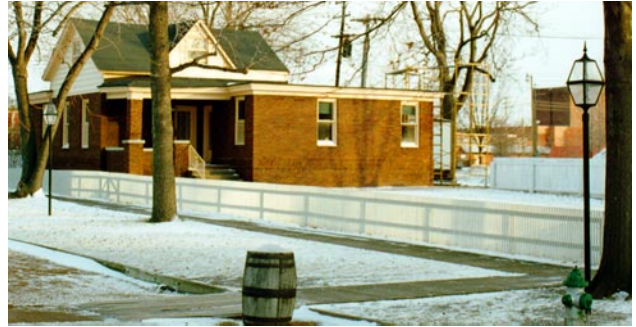
Pre-restoration, Charles Arnold House, Lincoln Home National Historic Site
