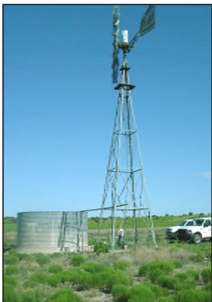
The Pueblo of San Felipe repaired and rehabilitated windmills, using NAAP funding.
