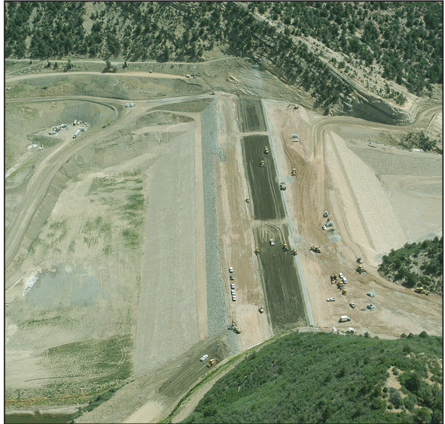
An aerial view of Ridges Basin Dam construction.
