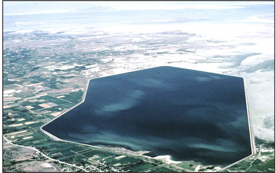
An aerial view of Watkins Dam.
