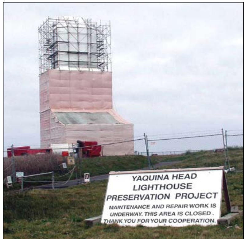
Figure 38. The BLM stabilized the Yaquina Head Lighthouse in Washington in 2007.
