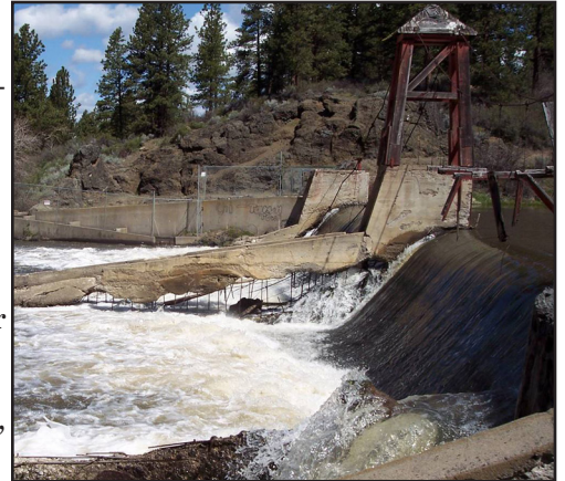
Built in 1914, Chiloquin Dam helped farmers in the Upper Klamath Basin irrigate their fields. Now irrigators will get water deliveries through a new pumping system. (USFWS photo)
