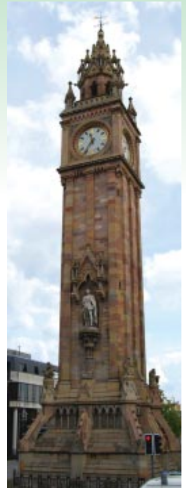
Below: Standing 113 feet tall, the Albert Clock in central Belfast is built on wooden piles on reclaimed land and is known as Belfast's "Leaning Tower of Pisa." The top leans four feet off the perpendicular.
