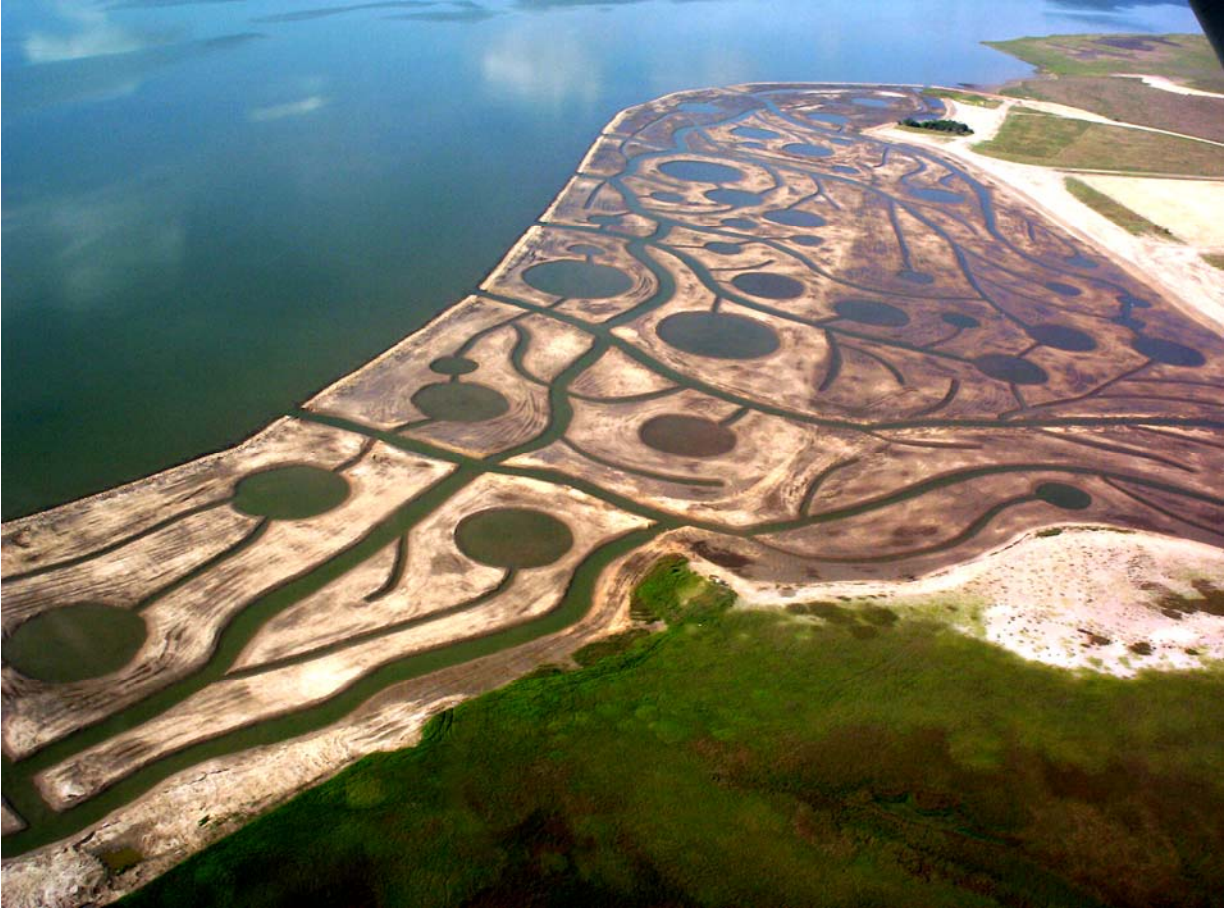
Constructed wetlands along the Texas Gulf Coast prior to revegetation
